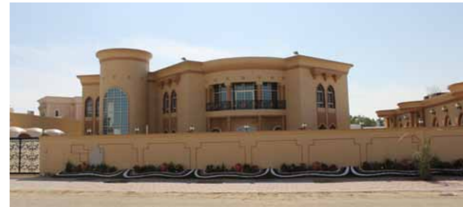
Extension in Villa on Plot No.281-1165 at Al Khawaneej-I
