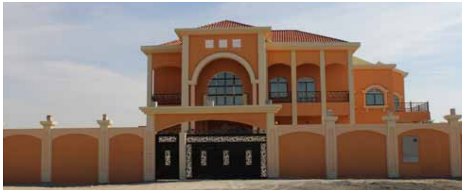
Villa (G+1) Villa on Plot No.263-1293 at Al Mezhar-II
